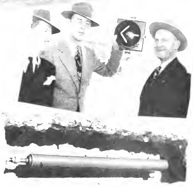
es at automatic traffic signal in San Diego. Top left—Electric brain that receives messages from magnetic traffic detectors and operates signals. Top right—Pedestrians on safety island awaiting effect of push button signal. Center—Market and Pacific intersection. Bottom left—Pedestrian "Wait-Walk" signal. Bottom right—Left turn signal and magnetic detector of buried pavement
